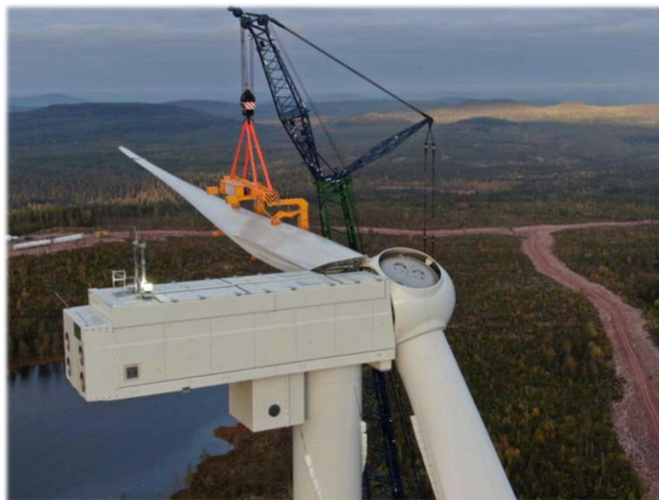
Figure 3.- 5.X Wind turbine generator assembly
