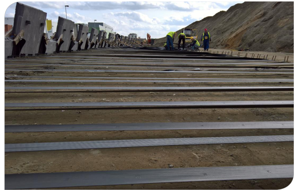
Paraweb used for soil reinforcement
