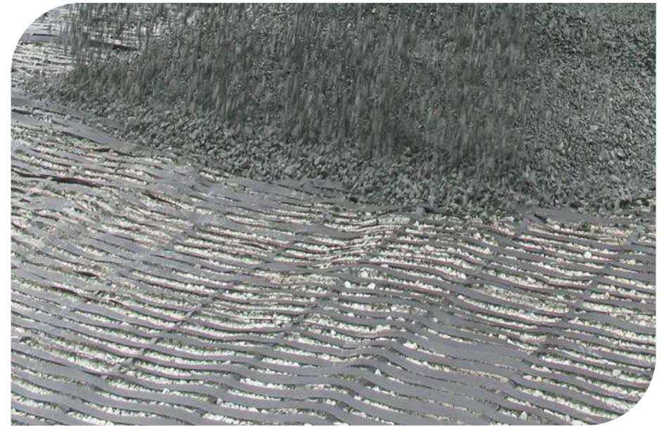
Installation of ParaGrid
