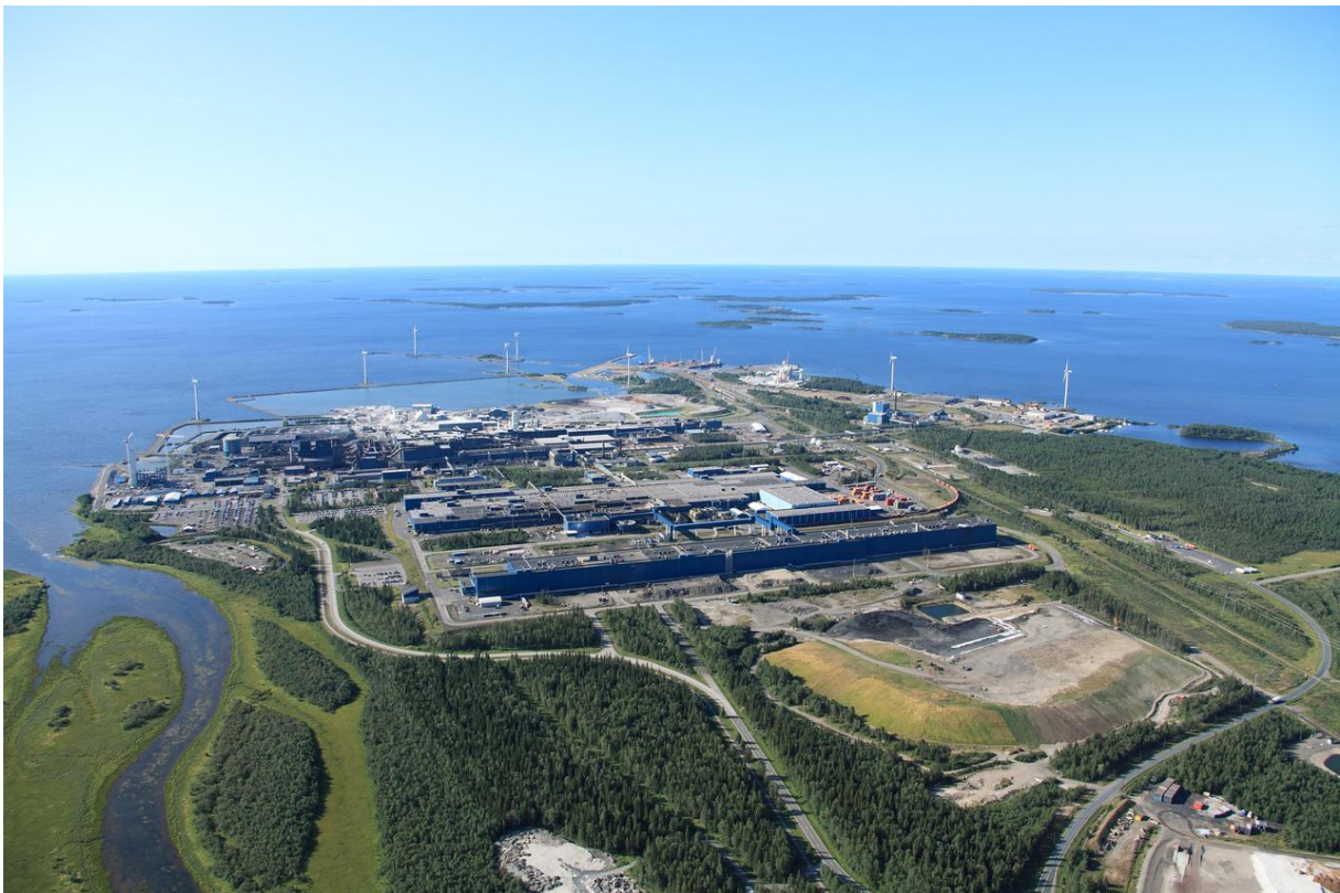
Figure 3 Ferrocrome is an integral part of Outokumpu's operations, and supported by our Kemi mine.
