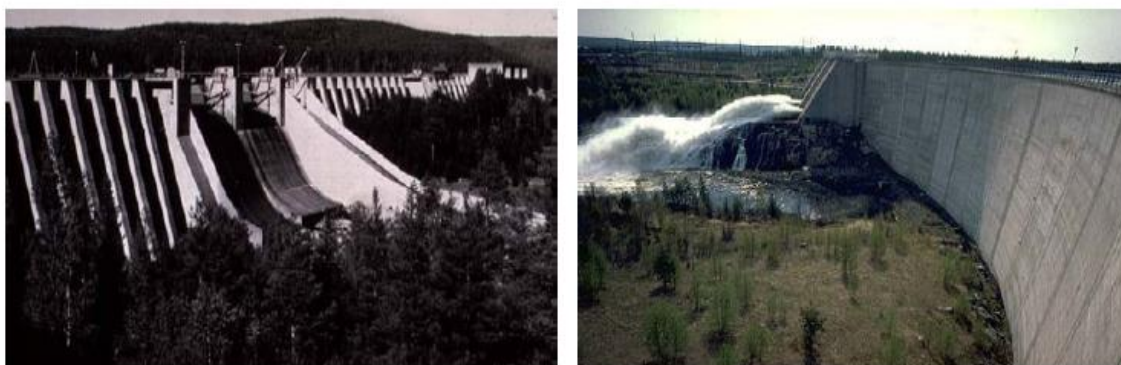
Figure 4 Downstream views of, on the left, a buttress dam and, on the right, an arch dam.
