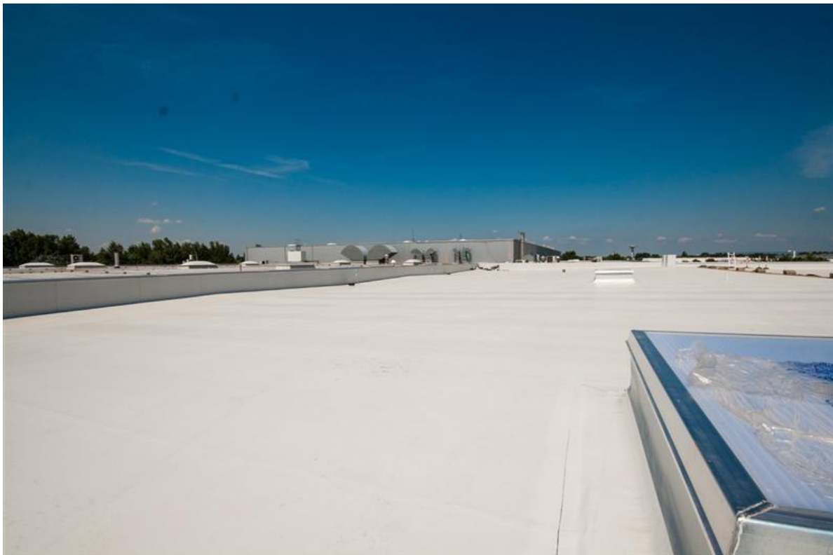
Figure 3: Membrane MAPEPLAN PLUS on fully exposed roof
