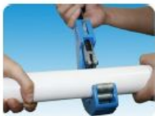
Step 1: Pipe cutting
