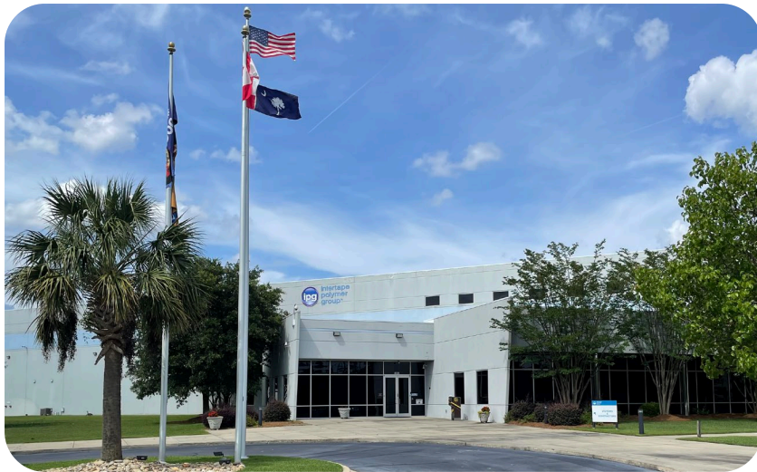
IPG Facility, Blythewood, South Carolina
