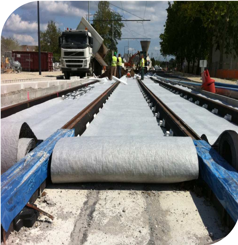
MacDrain W installation
