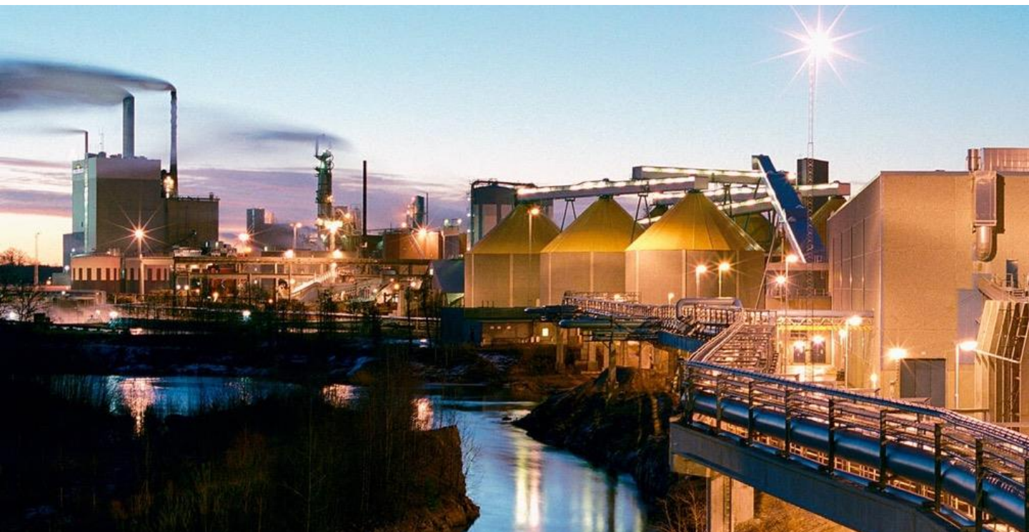
SKÄRBLACKA PM7 – THE PRODUCTION SITE FOR ConFlex Glaze WS
