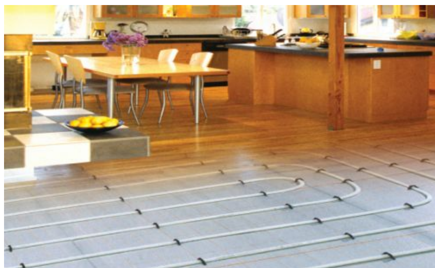
Figure 2- PE-RT piping diagram for heating application
