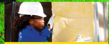
Cavitybatt Glasswool: An innovative dry wall insulation
