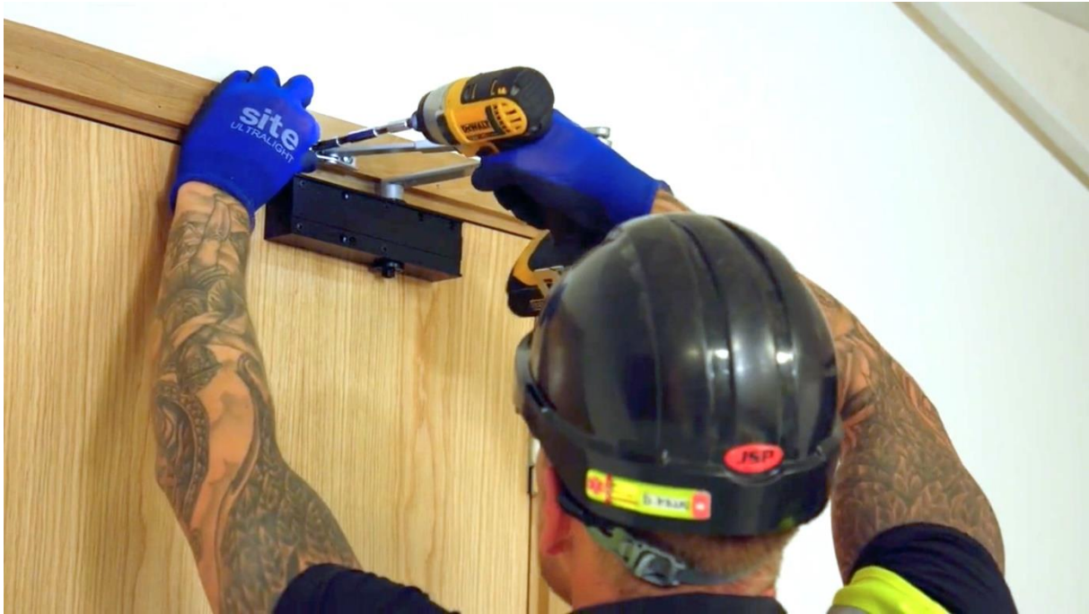
Figure 6: Generic example of installing ironmongery
