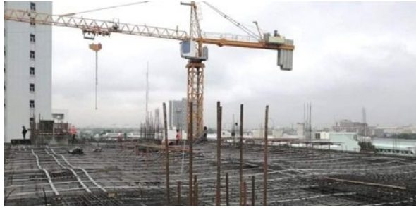
Bonded post-tensioned flooring system
