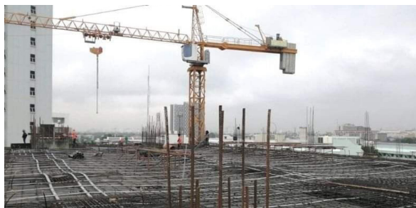
Bonded post-tensioned flooring system
