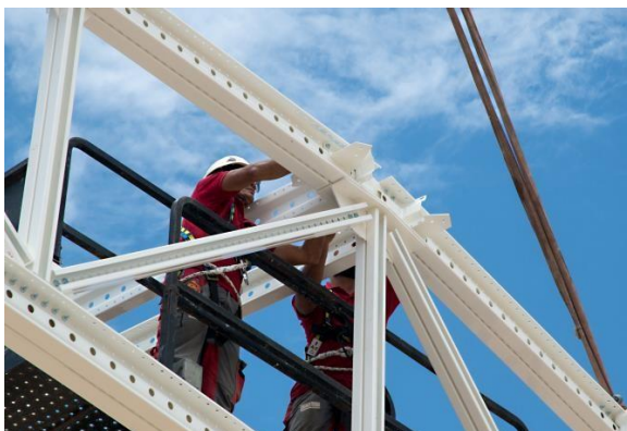
Figure 4: Installation of the Structura system
