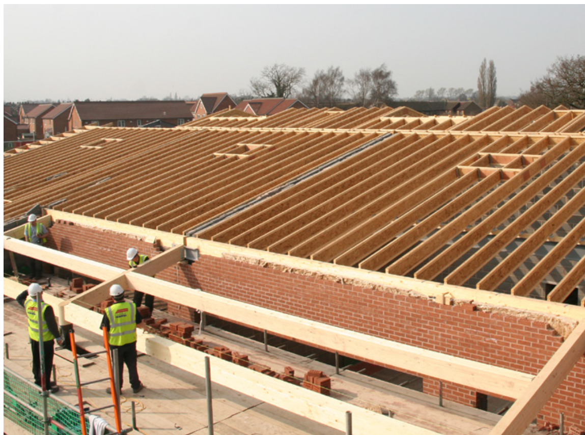
Figure 1: JJI-Joists in roof
