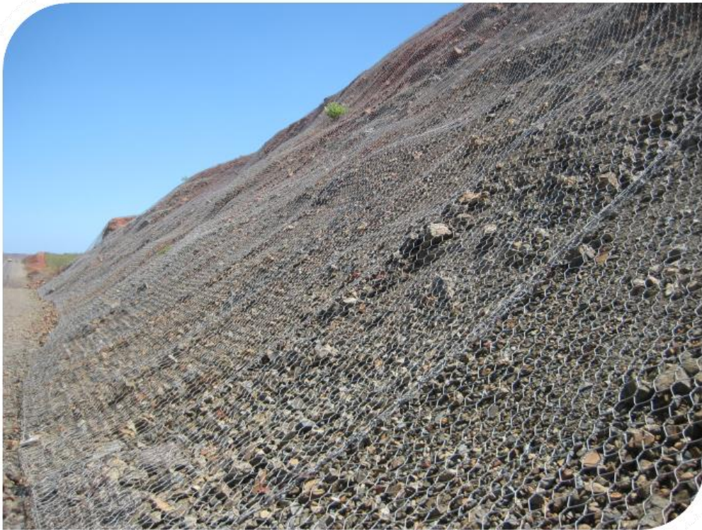
DT Mesh Netting installed for Rockfall Protection
