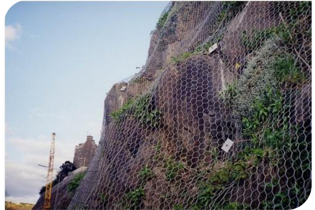
DT Mesh Netting installed for Rockfall Protection
