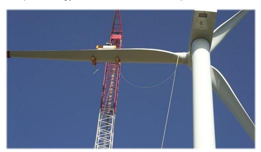
Figure 3: Wind turbine generator assembly
