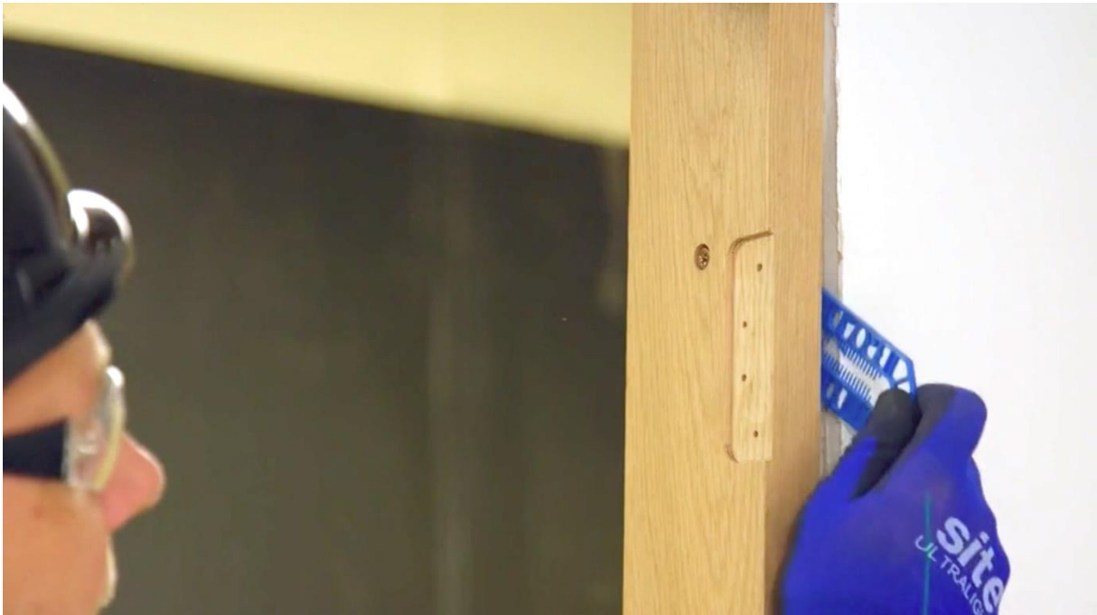
Figure 5: Generic example of install packer
