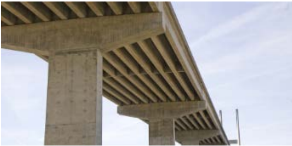
Pre-stressed concrete Girders
