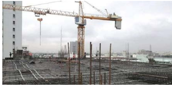
Bonded post-tensioned flooring system
