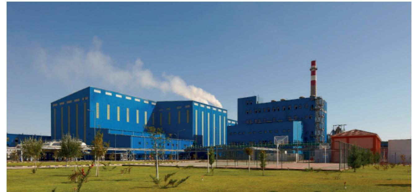
Eti Soda was the first facility in the world to utilise innovative solution mining technology on a commercial scale and has almost 25 years of remaining mineable trona reserves. The production plant consists of three sub-units: mining, processing and a coal-powered cogen facility producing power and steam for use in the plant. The plant was designed and engineered by TCC and CMEC, and utilises Siemens and Goulds rotating equipment and control systems.
