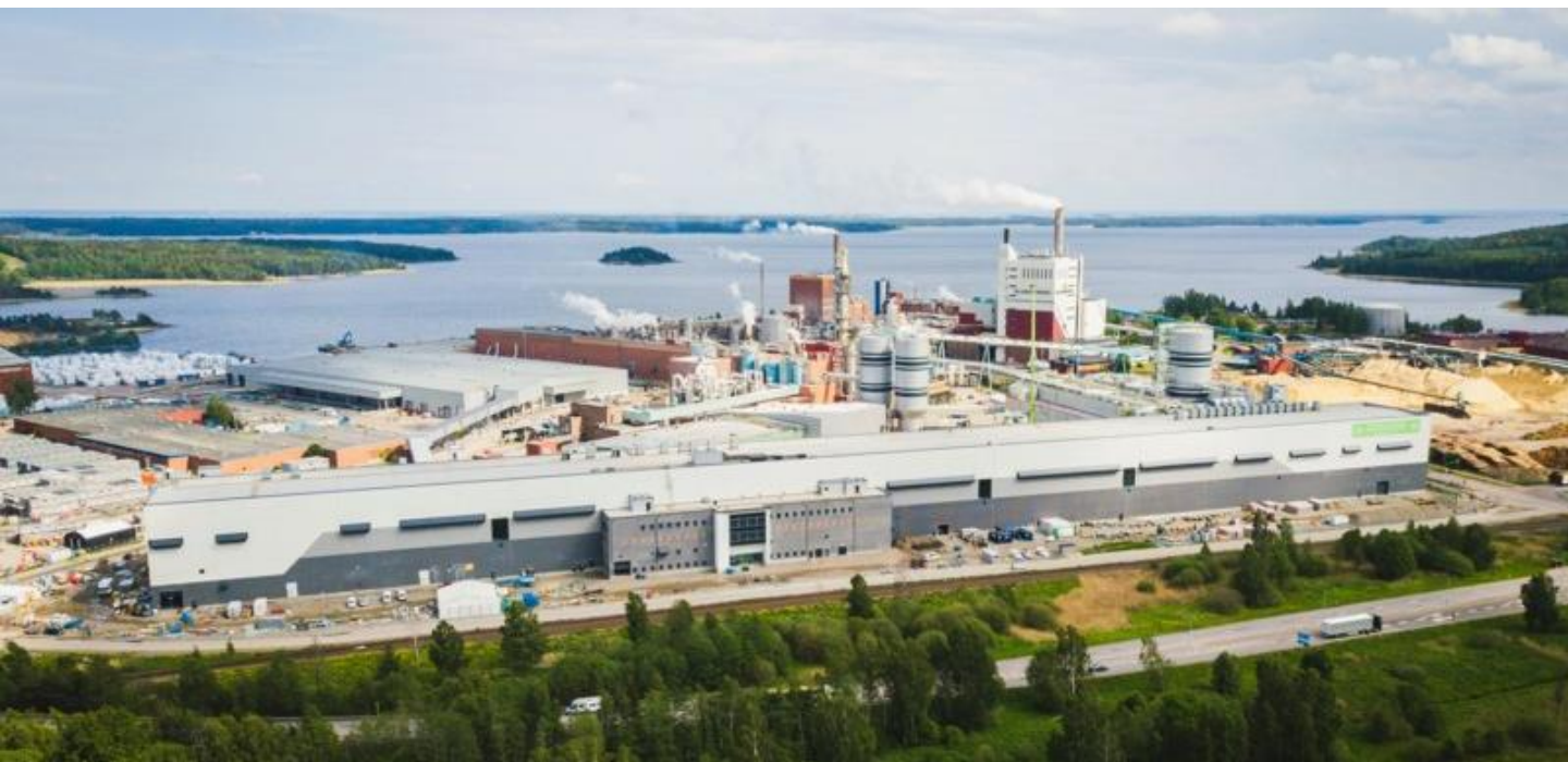
GRUVÖN – THE PRODUCTION SITE FOR CROWNBOARD PRESTIGE 290
