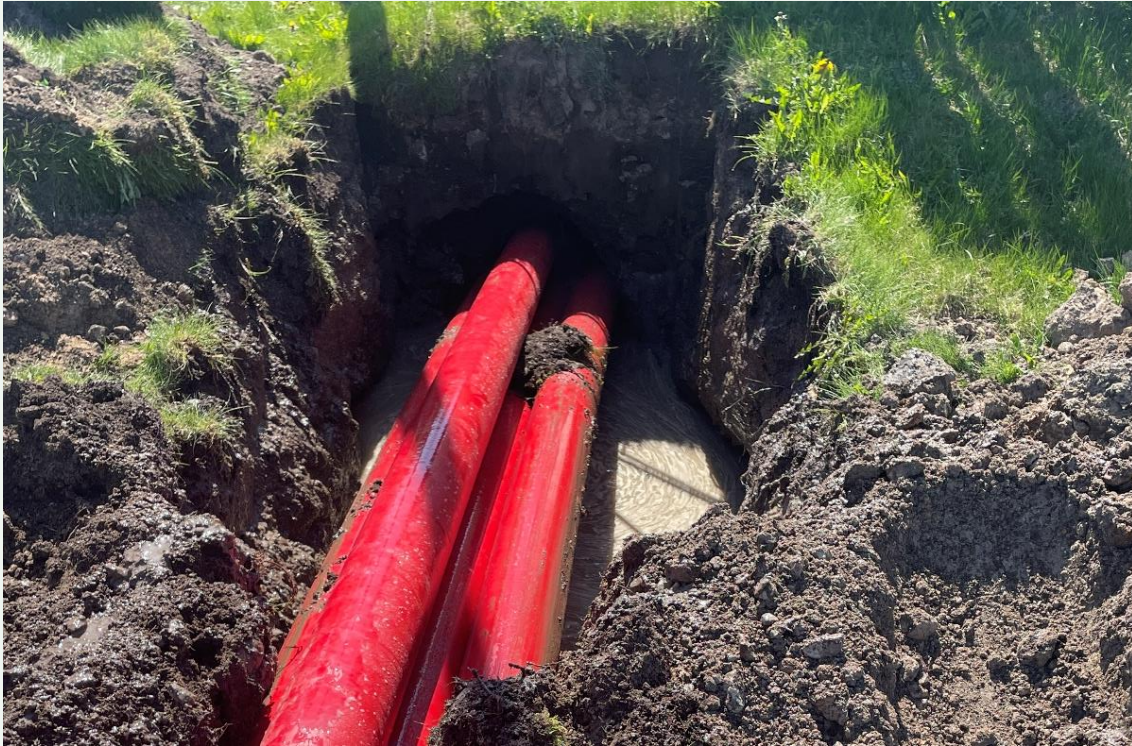
Figure 1. Cable protection pipe installation
