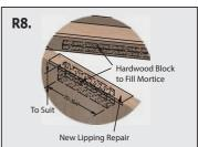
R8. Concealed closer mortice reinstated Maximum size timber (640Kg/ m3): leaf closer body infill; L 338mm x H 47mm x W 35mm. Lipping; L 575mm x H 8mm x W44/54mm. Frame slide arm infill; L 448mm x H 22mm x W35mm.
