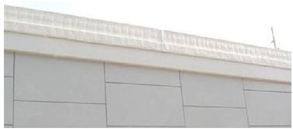
Concrete panels for pre - cast segments
